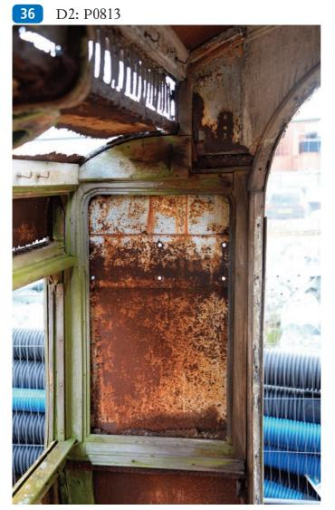
Above and right: Joinery at upper corners, showing the interior of a window, the window ledge, and mirror frame fitted either side of the doorways.
