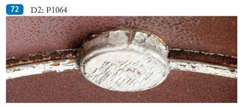
All ten interior lamps had metal housings mounted on wooden roses. On no.163 one of the ceiling roses was blanked off. The other blanking sheet was missing from the rose, exposing the wiring. See also Ref 110.
