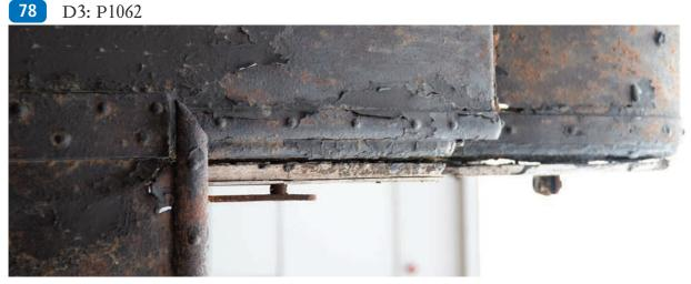
Seen from above, at the left is the edge of the canopy with the upper curved roof in the middle and the lower curved roof to the right. The teak mouldings above the doorway and metal upper door runner may also be seen.
