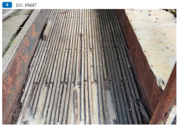
Wooden slats fitted on top of lito-silo base above a corrugated metal floor. (Lito-silo is a pseudo concrete largely composed of whiting, cork dust, iron oxide and cement.)
