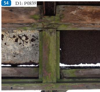
Joinery where two advert frames meet. The contoured structural flitched beam supporting across the clerestory roof above may also be seen emerging from the horizontal upper wooden framework.
