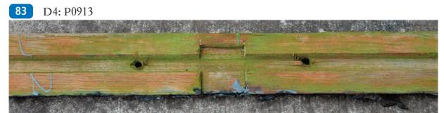
A short section of teak moulding, flipped about its horizontal to show the vertical rebate for the roof strap. A horizontal channel was seen on all other similar mouldings removed.
