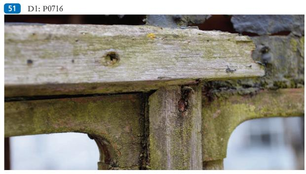
Bevel-edged teak moulding at junction of horizontal and vertical flitched beams at window tops.
