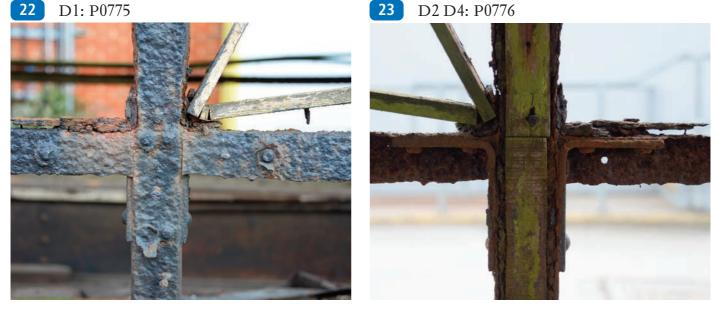
Above: The internal square brackets can be seen securing the continuous vertical to the horizontals abutting either side. Very rusted metal fillets were apparent on all four sides between the window frames and flitches. Right: The same joint from the inside.
