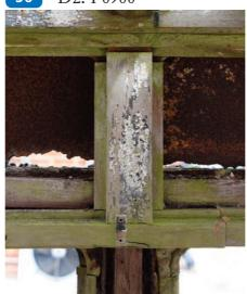
Vertical advert panel separators were held in place top and bottom by mortise & tenon joints.
