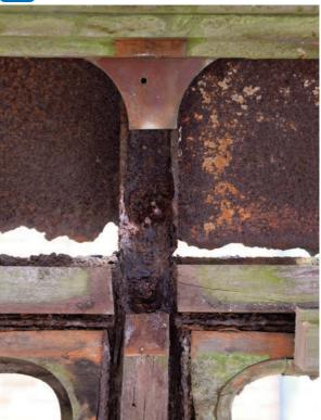
With the vertical joinery removed the arrangement of the horizontal and vertical teak inserts are revealed; the shaped rear metal plate may also be seen.
