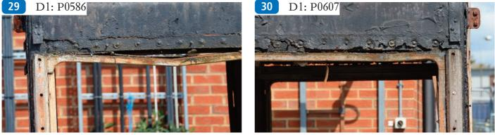
There was evidence of metal fillets between the flitched beams and all four outer edges of the window frames, though their purpose remains undiscovered. When mouldings were in place these were not visible.
