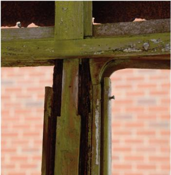
Interior where the overhead 13/4-inch beam projects below the upside-down horizontal 'L'-shaped beam and sits inside the 2-inch flitched vertical beam. The vertical teak insert may be seen rebated to receive the roof beam. 63 D2: P0934
