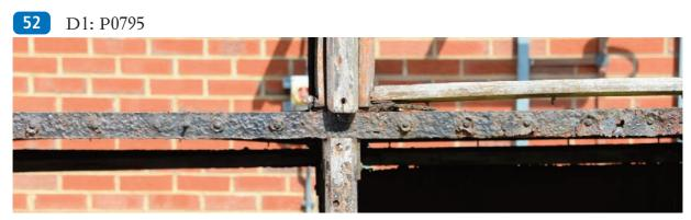
Vertical teak moulding showing mitres with (missing) horizontal.
