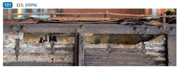
The north end of the underside. The rusted corrugated steel floor has exposed the lito-silo.
