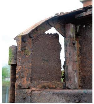
The carriage is on its side and the under-seat plate therefore to the right vertically here. At the top of the picture a three-dimensional bracket is holding the north side panel (to the right of its doorway seen from outside) to the 'L'-shaped corner vertical and lower 'L'-shaped horizontal flitched beam. The two horizontal teak inserts have been rebated to clear the bracket.
