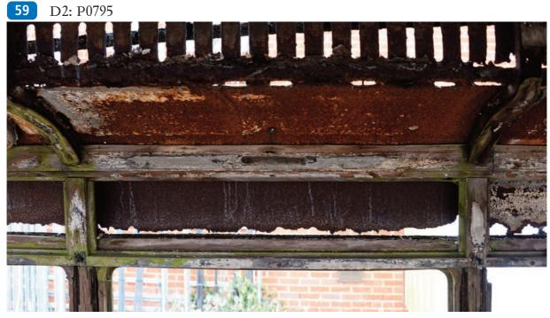
A complete advert frame, also showing the inside of the external roof panelling, severely rusted along its bottom edge. The top of the upside-down 'L'-shaped beam may be seen outside.
