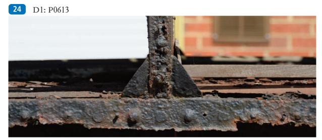
The three-dimensional brackets, one each side of the vertical, above, seen from exterior and below, as seen from interior.
