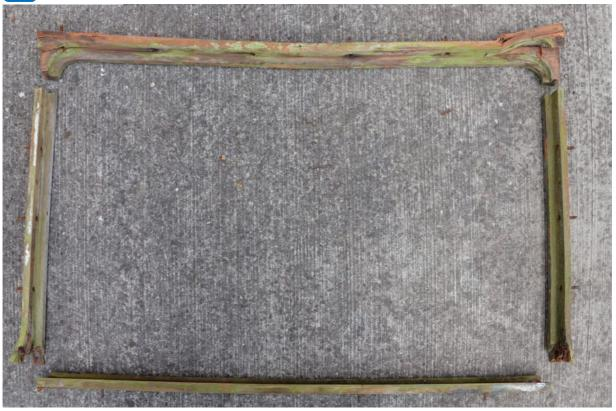
Interior of a removed window frame. All four sides of the wooden frame were rebated to receive the 1/4-inch plate glass, with an internal wooden bead securing it all round. Strips of leather were in place, either side of the glass, within the resulting groove formed by the outer frame and the inner beading.
